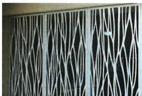
Material tag: SS-01 Element: EXTERNAL WALL PODIUM CARPARK Finish: POWDER COAT - "NATURAL SILVER 7365K DURATEC X15" OR SIMILAR
