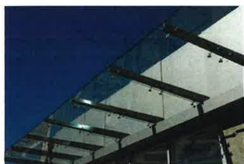
Material tag: AW-01 Element: HOTEL AND RETAIL AWNING Finish: "DULUX - MICACEOUS IRON OXIDE" OR SIMILAR & TRANSPARENT GLASS WITH WRIT WORK
