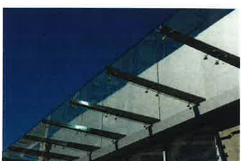
Material tag: AW-01 Element: HOTEL AND RETAIL AWNING Finish: "DULUX - MICACEOUS IRON OXIDE" OR SIMILAR & TRANSPARENT GLASS WITH FRIT WORK
